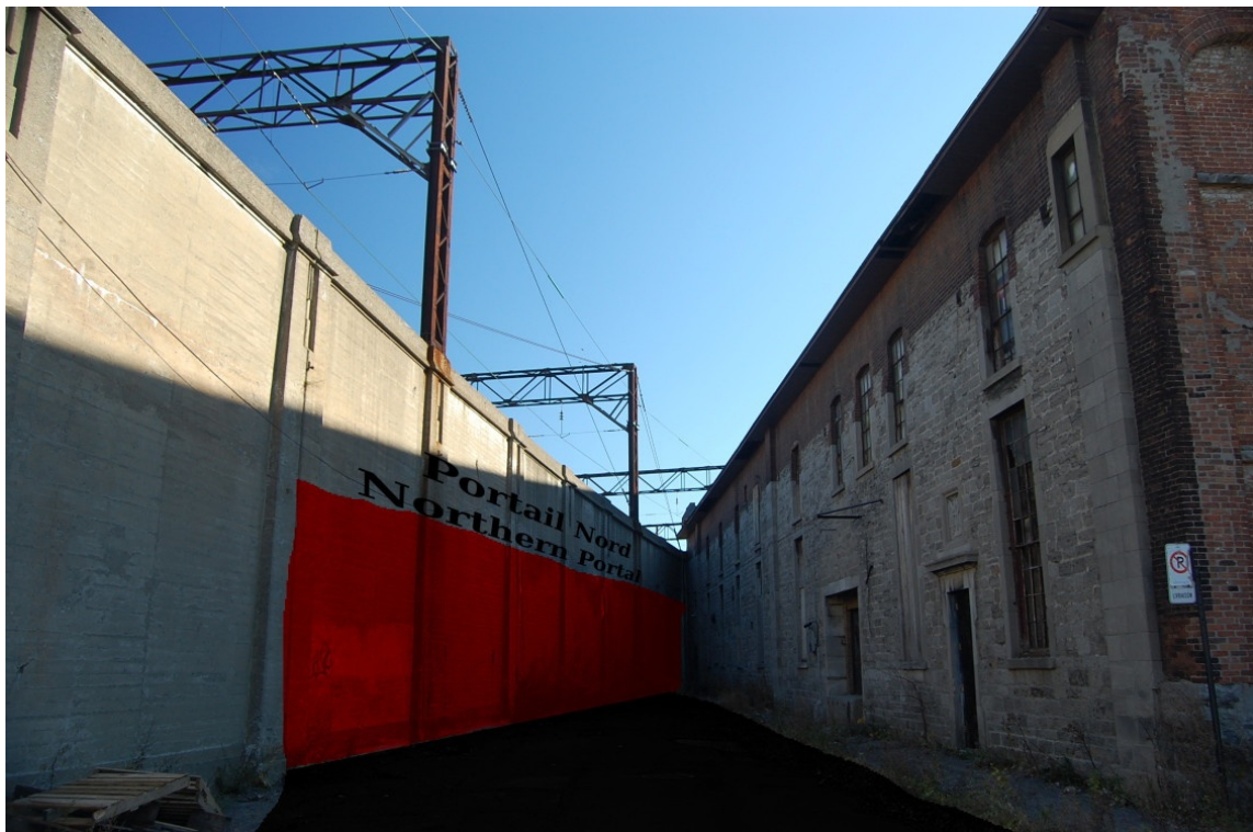
Figure 2. Northern Tunnel Portal and its extreme proximity to the historic New City Gas Co. (1847)
