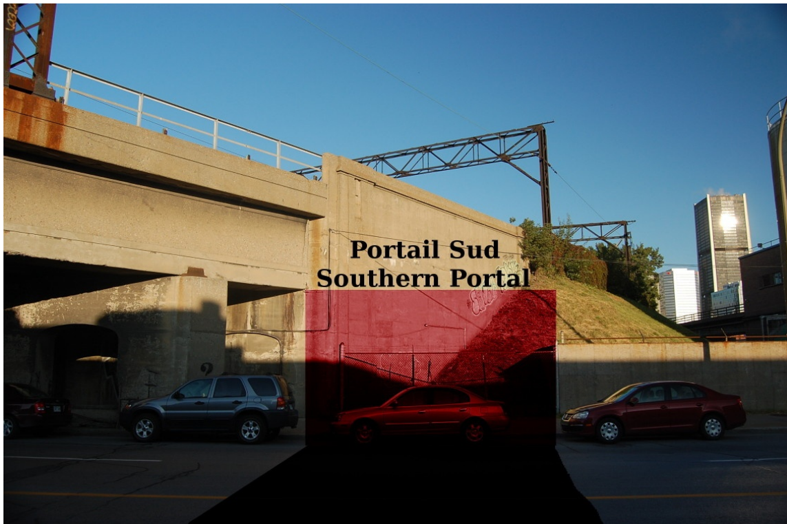
Figure 1. Southern Tunnel Portal and the dangerous blind intersection with Wellington St.
